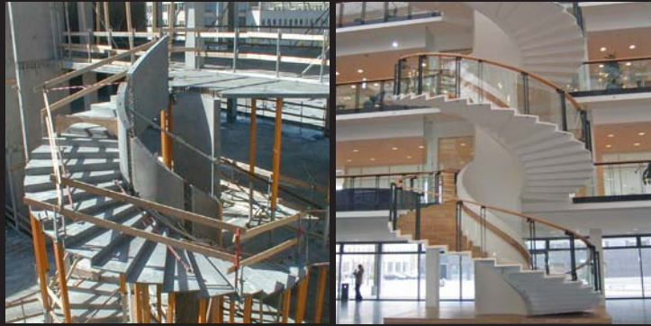
Individual elements are joined into a complete stairway – which appears as cast in one operation.
