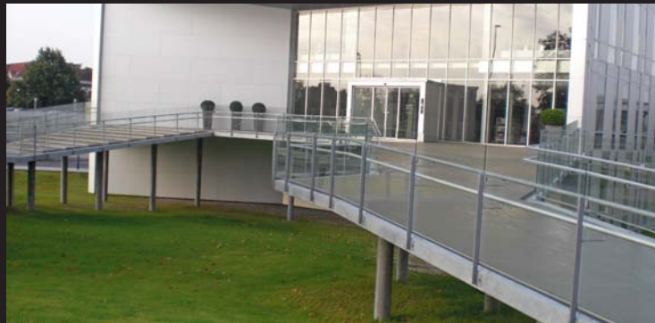
Combined stairway and ramp in front of Roskilde town hall, Denmark, is an example of a building made with elements that otherwise would have been casted in-situ. With CRC ® JointCast, the element solution resulted in a faster and more cost-effective construction and a much better quality.
