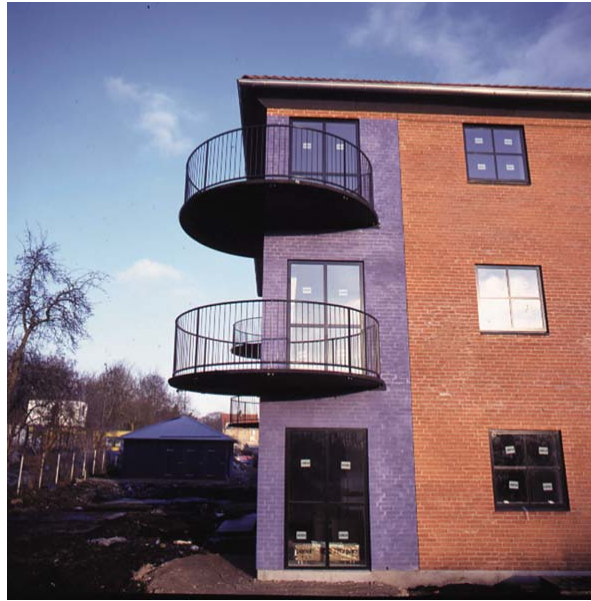
Figure 1 Cantilevered balcony slabs produced in a dark CRC.
