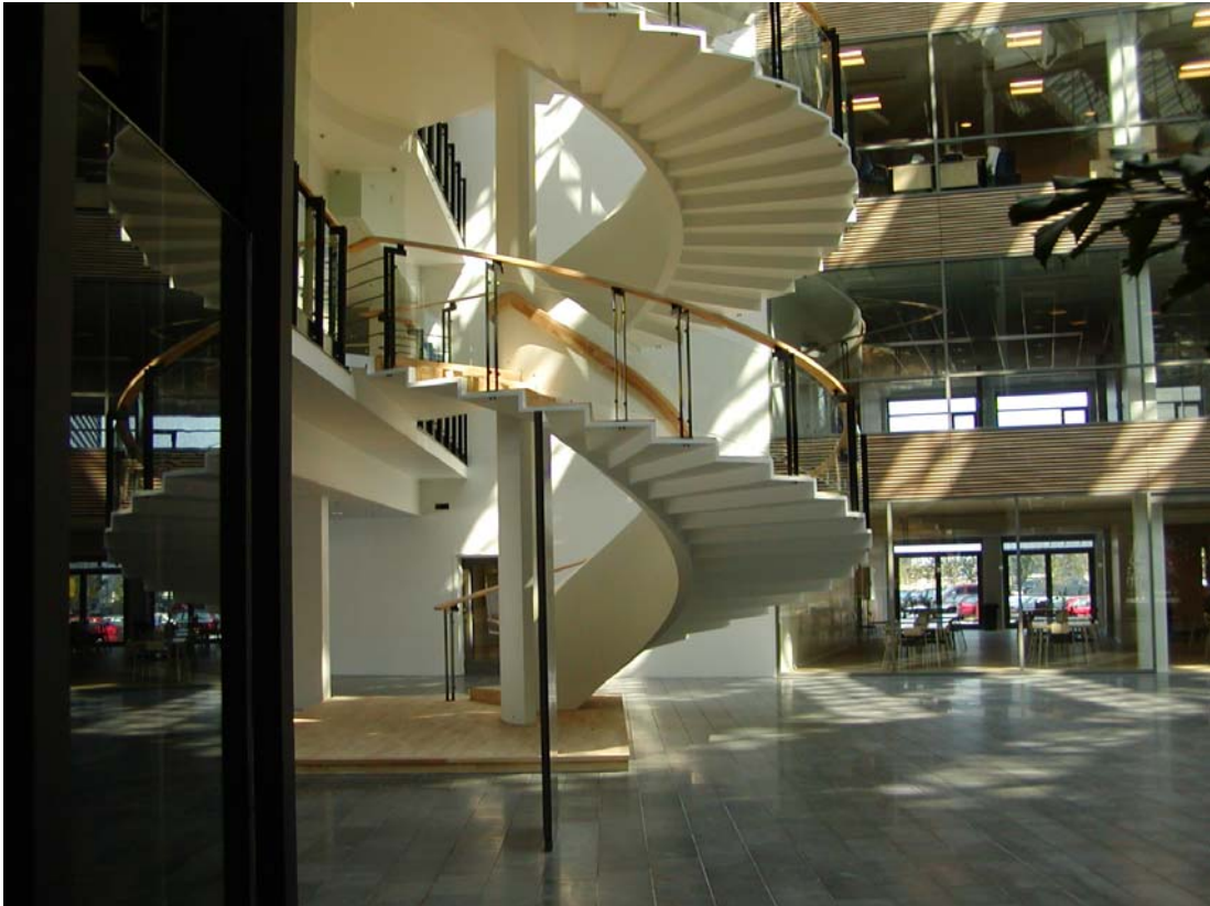
Figure 2 Spiral staircase with cantilevered steps produced in CRC.
