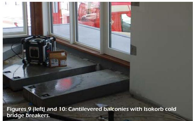
Figures 9 (left) and 10: Cantilevered balconies with Isokorb cold bridge breakers.
