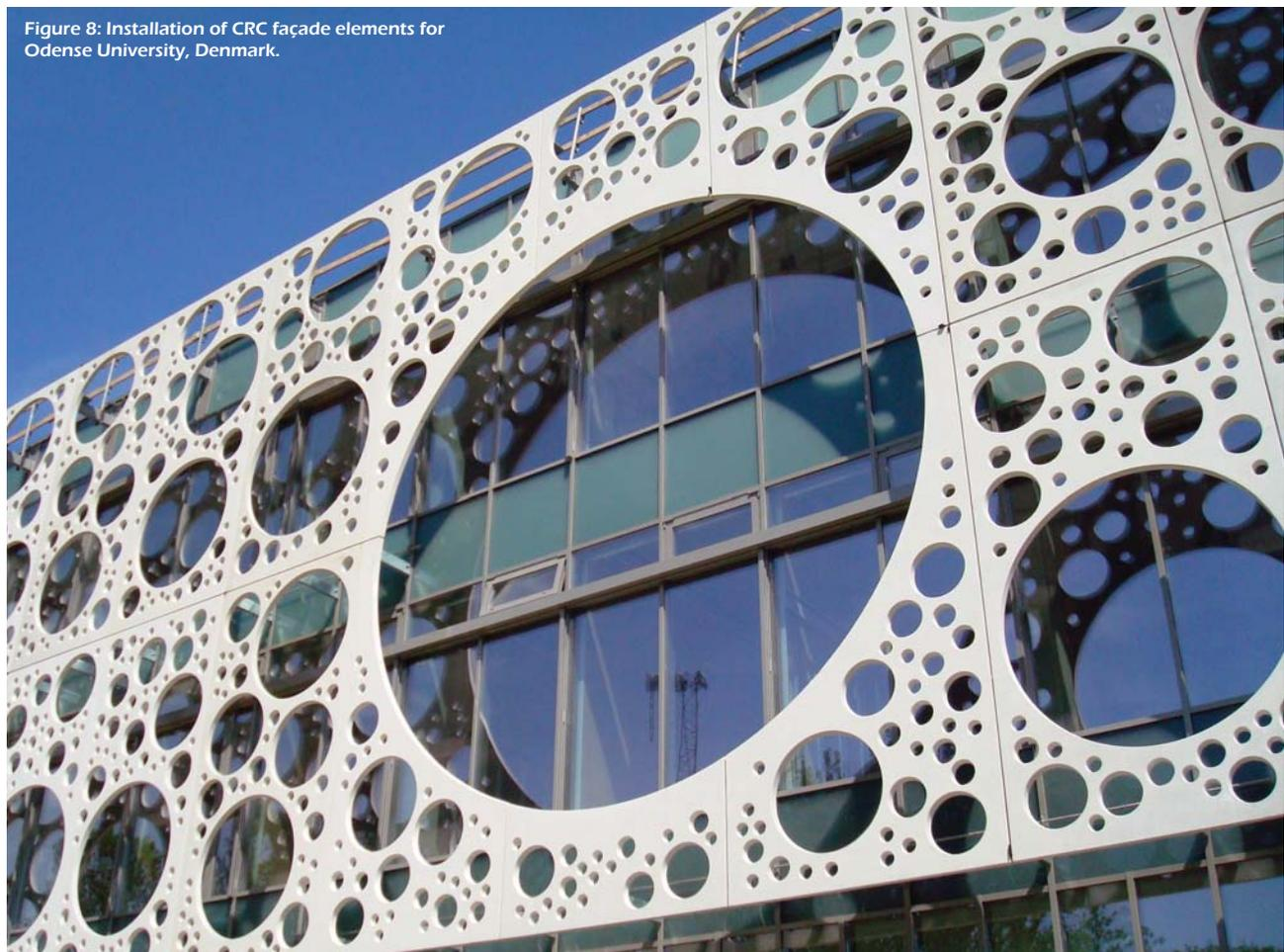
Figure 8: Installation of CRC façade elements for Odense University, Denmark.
