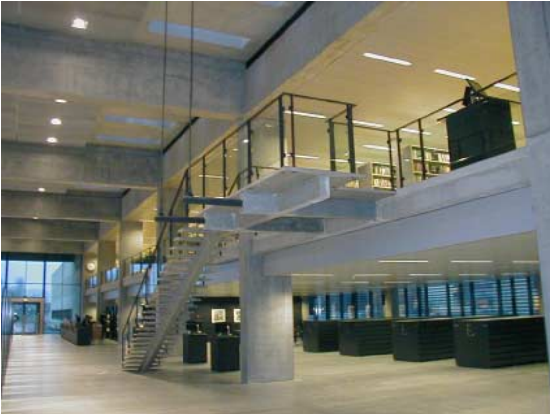
The staircase at the library of Roskilde University. The joint shown on the previous page is not visible and the beams crossing underneath the platform could have been cast on site.
