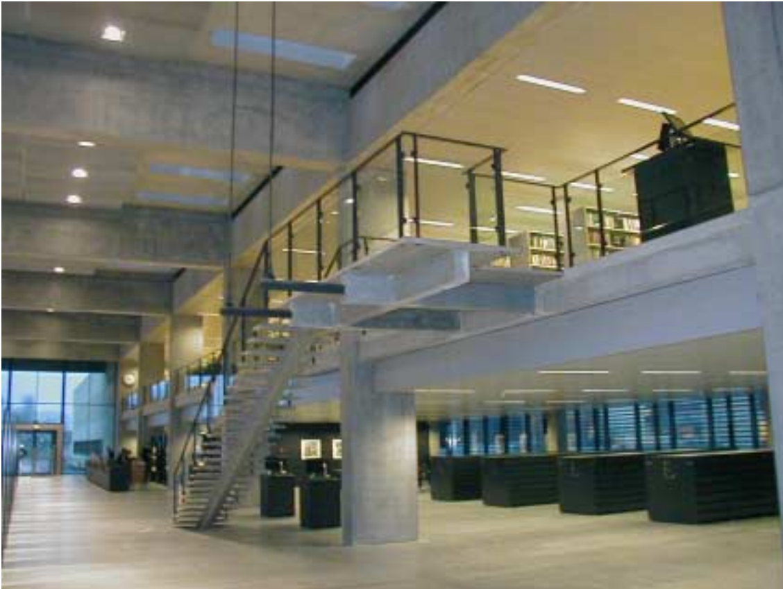
The staircase at the library of Roskilde University. The joint shown on the previous page is not visible and the beams crossing underneath the platform could have been cast on site.
