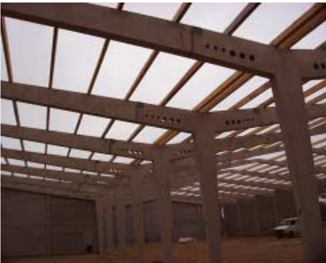
Joints for frames at Sdr. Felding. The joints were used to make the elements easier to transport.
