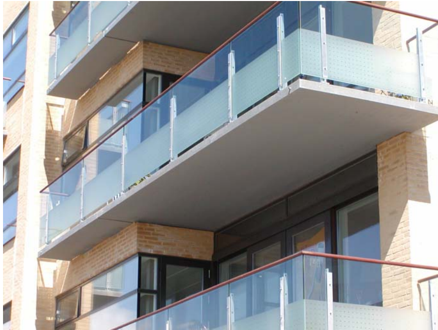
Figure 3 Cantilevered balcony slabs in CRC.
