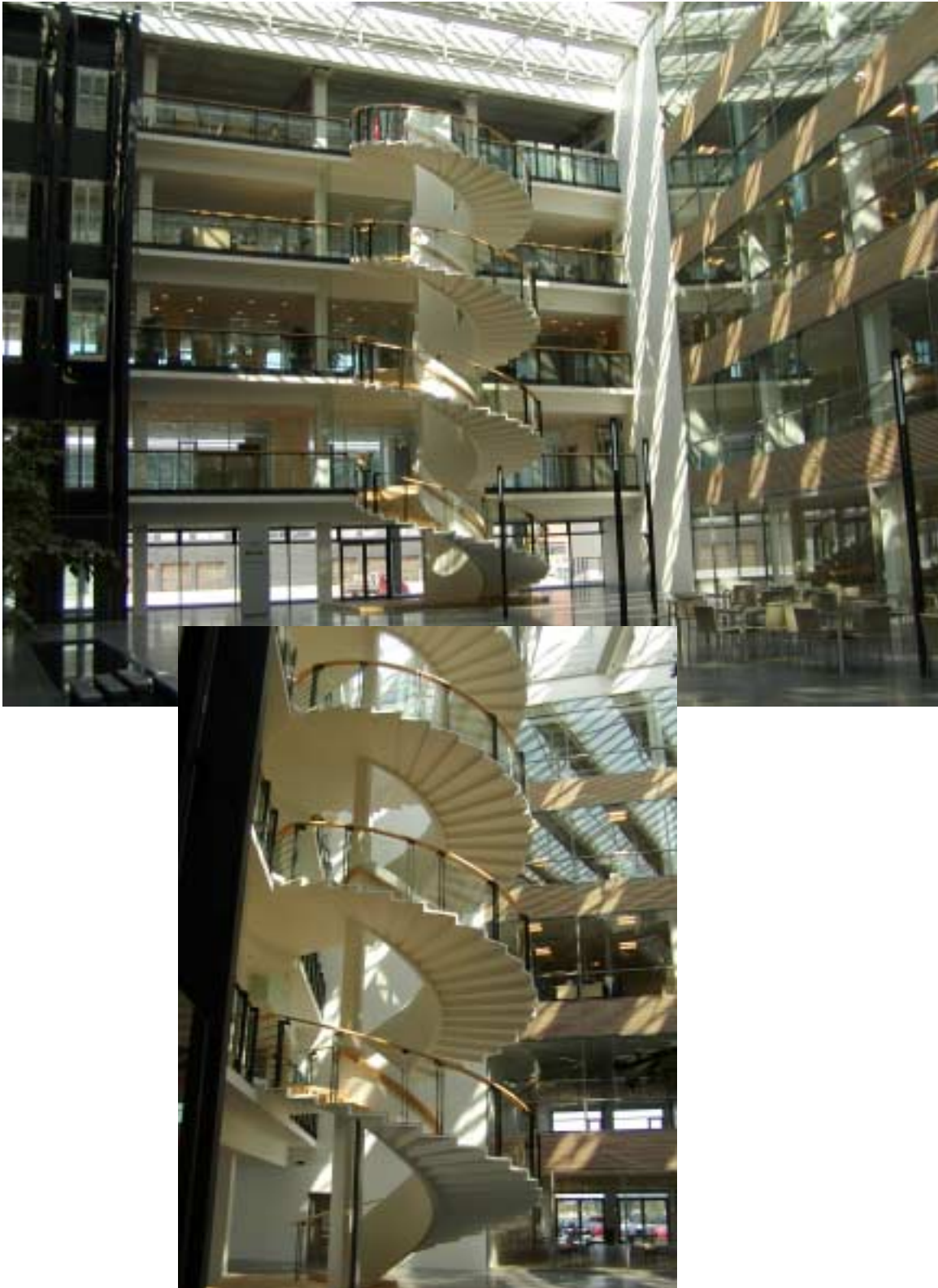
Spiral staircase in CRC produced as elements connected using CRC JointCast. The steps are cantilevered from the inner banister – a CRC beam which carries a lot of torsion. Architects are Arkitektgruppen Århus.
