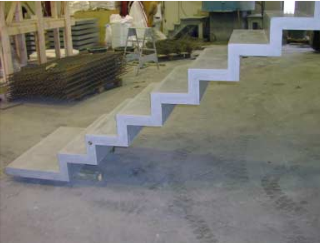
Staircase for the new offices of architects Arkitektgruppen Århus. There are no supporting beams for the staircase, the load is carried by the steps.
