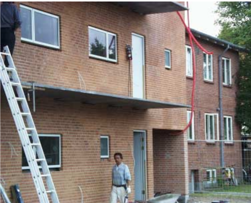
Cantilevered slabs being put in place in Silkeborg, Denmark.
