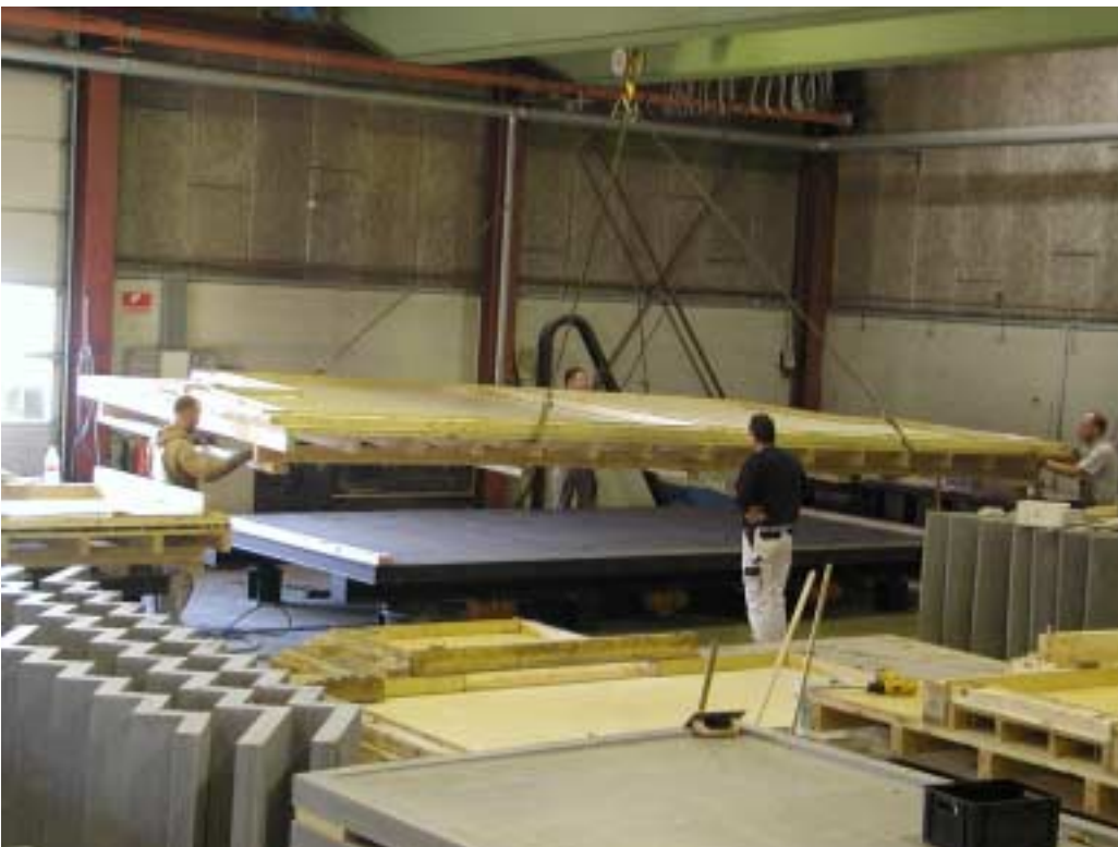
Formwork for balcony slabs being placed on one of the vibration tables at Hi-Con.
