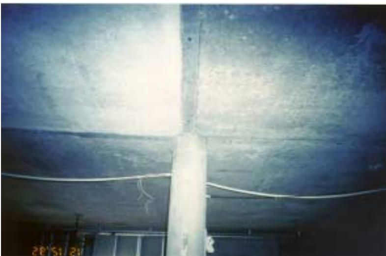
Pictures showing CRC JointCast used at Aalborg University. The 100 mm wide joints are stronger after 3 days than the slabs, which means that failure will never occur in the joints.
