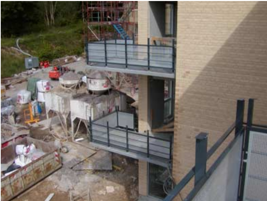
The balcony slabs at Sandegraven, Vejle at different stages of installation. The installation process is quite simple, as the “flaps” are bolted to the floor.
