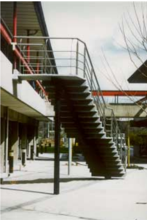
Staircase at Aalborg Portland A/S. Beam produced in dark CRC and steps in lighter CRC.
