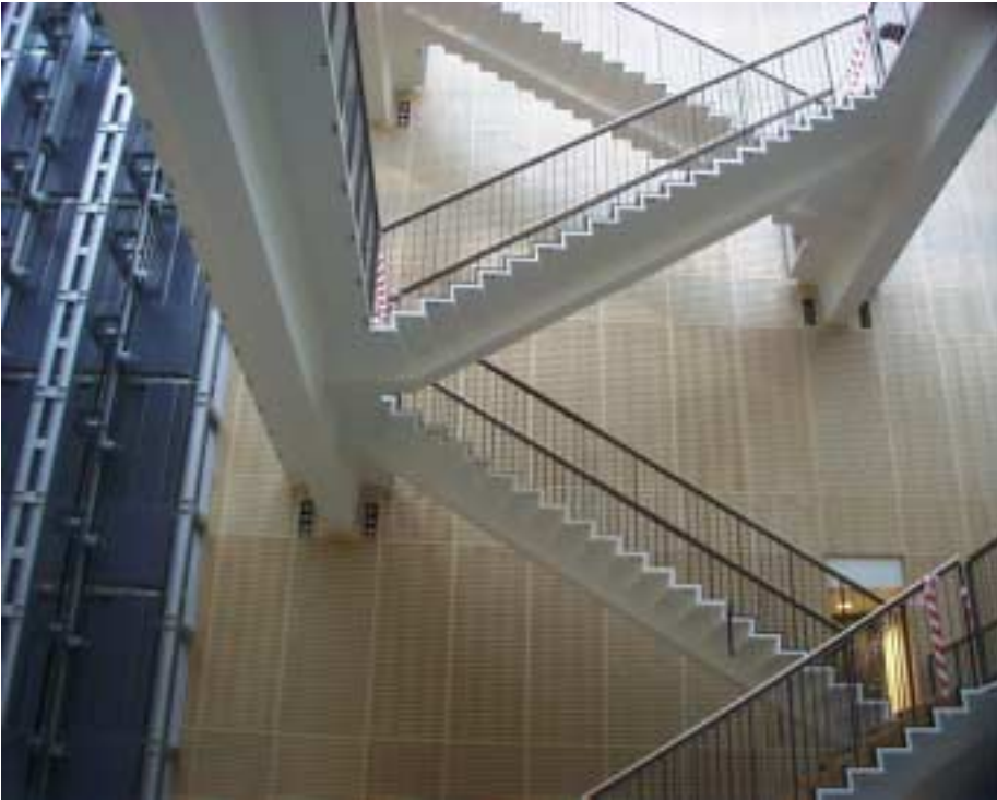
CRC staircase and walkways in Århus, Denmark designed by 3XNielsen.
