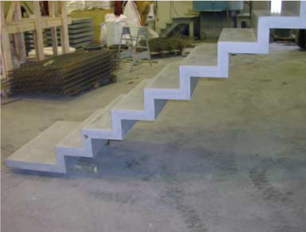
Staircase for the new offices of architects Arkitektgruppen Århus. There are no supporting beams for the staircase, the load is carried by the steps.
