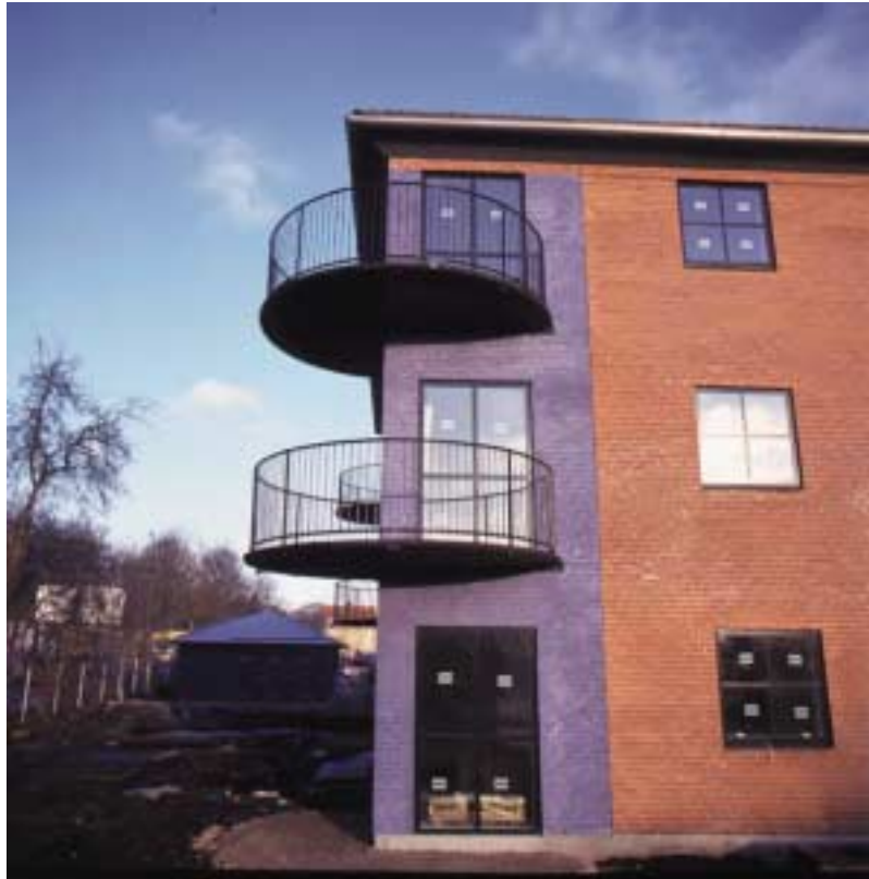
Photo 1 Cantilevered balcony slabs in CRC.
